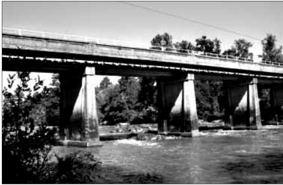
The water pipe beneath Bynum Bridge ultimately saved it.
